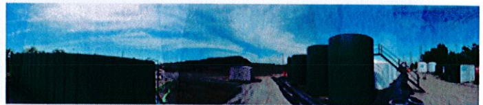
Image 2 - View from Left to Right: Raw Storage Tanks (20,000 Gallons); Shed; 10 x 15 Steel Tanks (8,400 Gallons); 10 x 10 Poly Tanks (8,100 Gallons)
