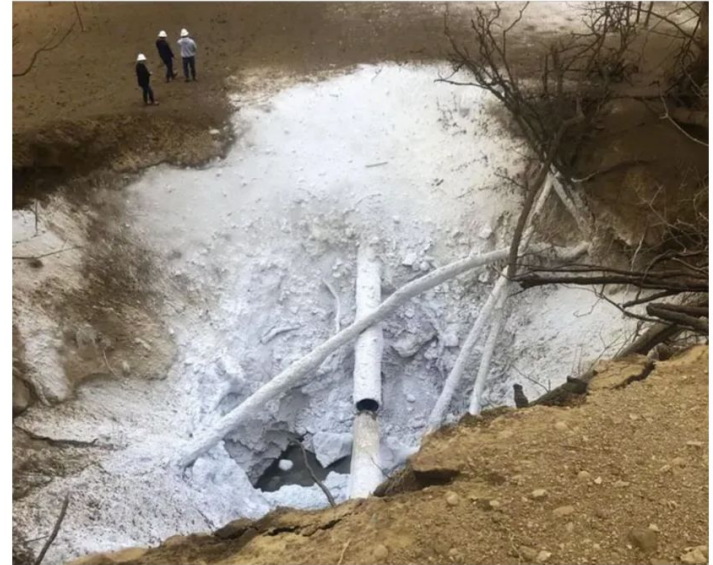
This photo shows the spot where a carbon dioxide pipeline ruptured in Satartia, Miss., in February 2020, leading to the evacuation of 200 residents and the hospitalization of 45 others. No one was killed. Yazoo County Emergency Management Agency / Submitted
